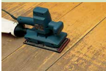
To renovate a floor the lacquered surface must be first sanded.
