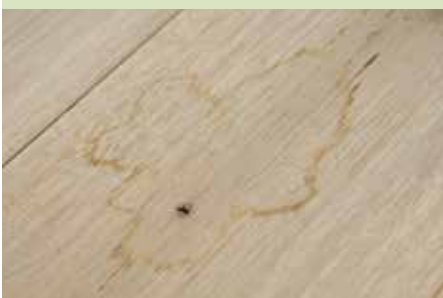
Due to poor resistance against liquids an unsightly water stains can quickly develop.
