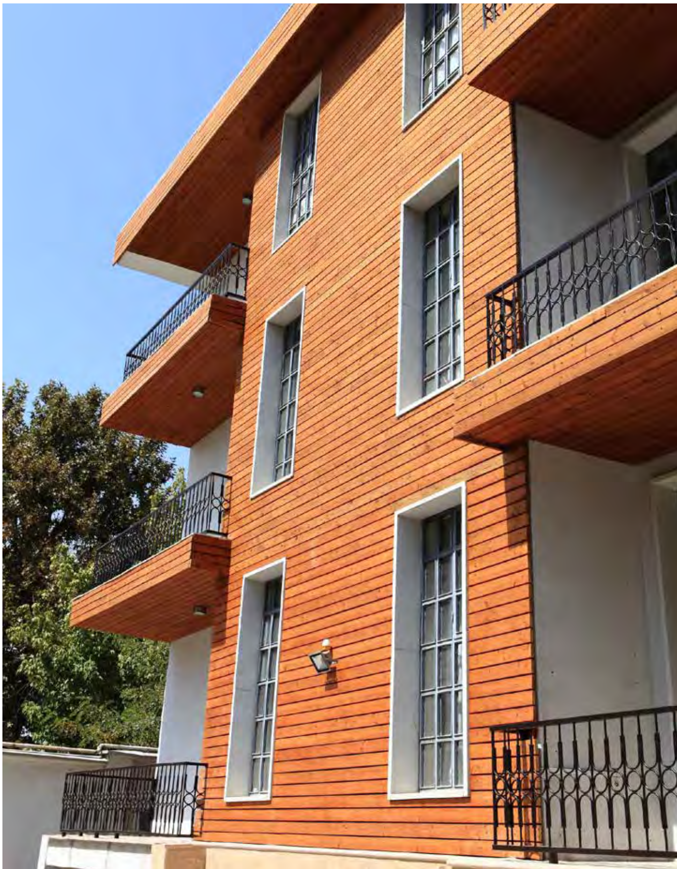
REAL FACADE, Thermo pine, Raute profile 26 x 92 mm, left natural
