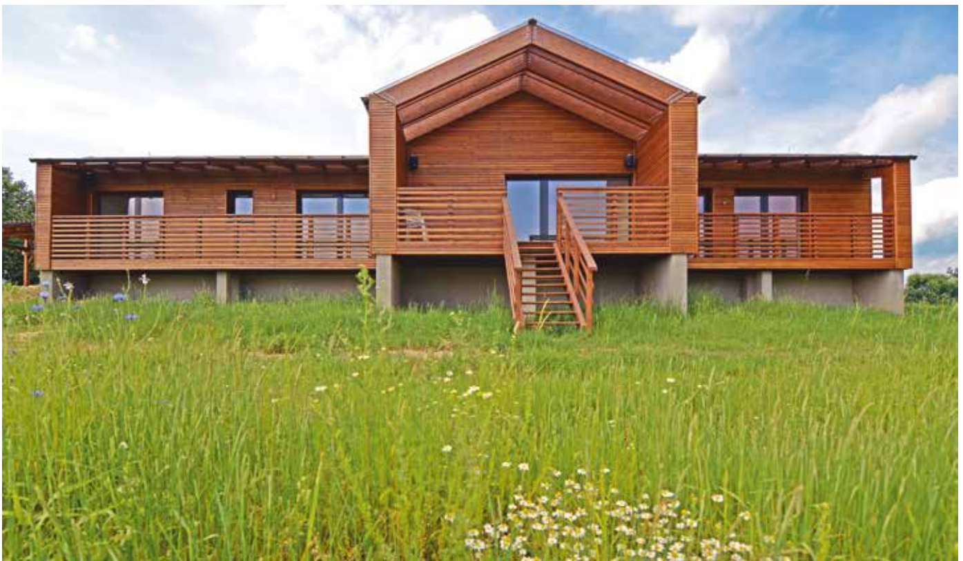
Siberian larch facade, Raute profile 28 x 68 mm, surface treatment OSMO – UV Protective oil n. 420 transparent, 3 years after application
