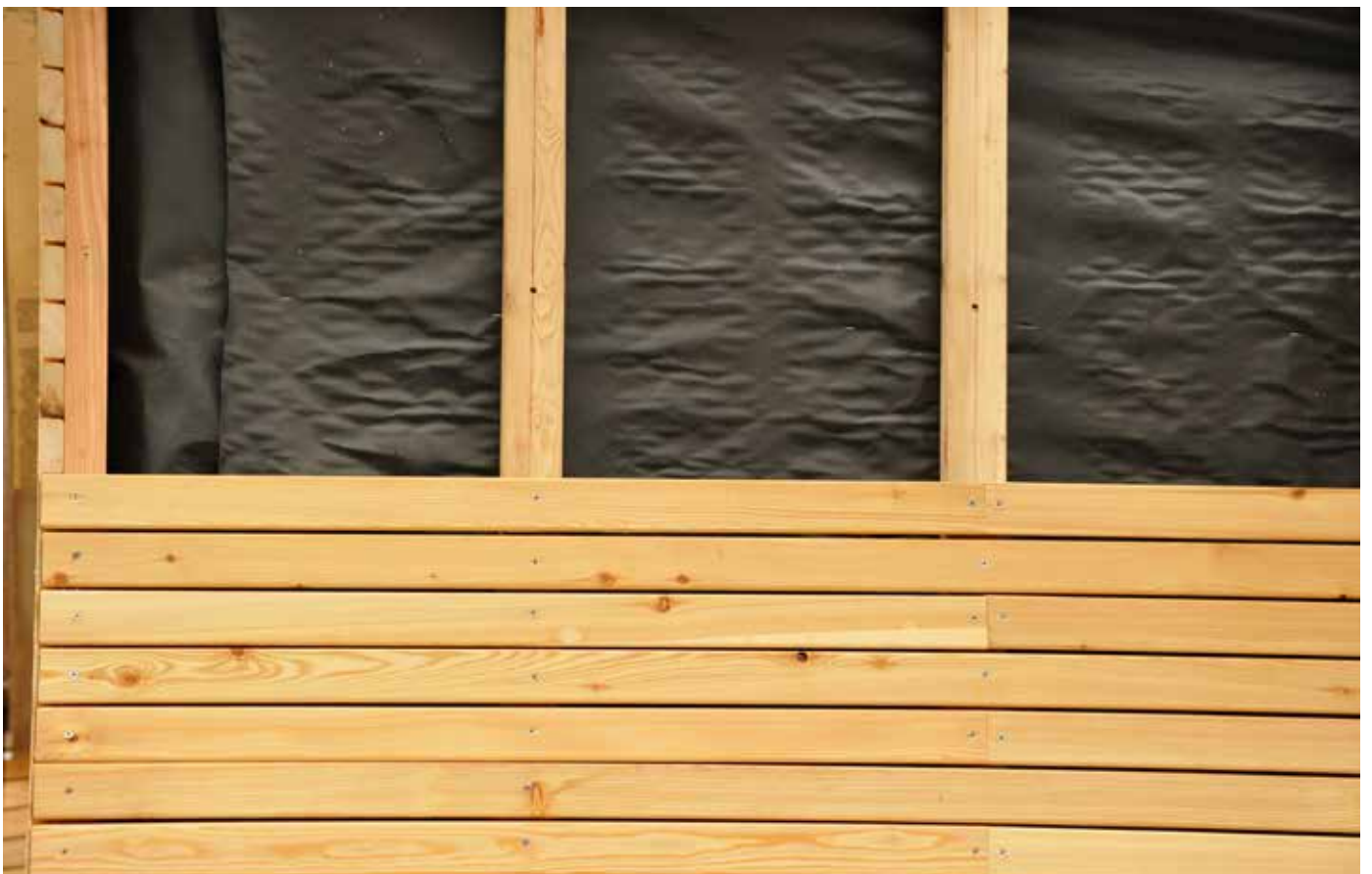
Installation of Raute profile 28 x 68 mm, ventilated facade with the use of diffusion foil
