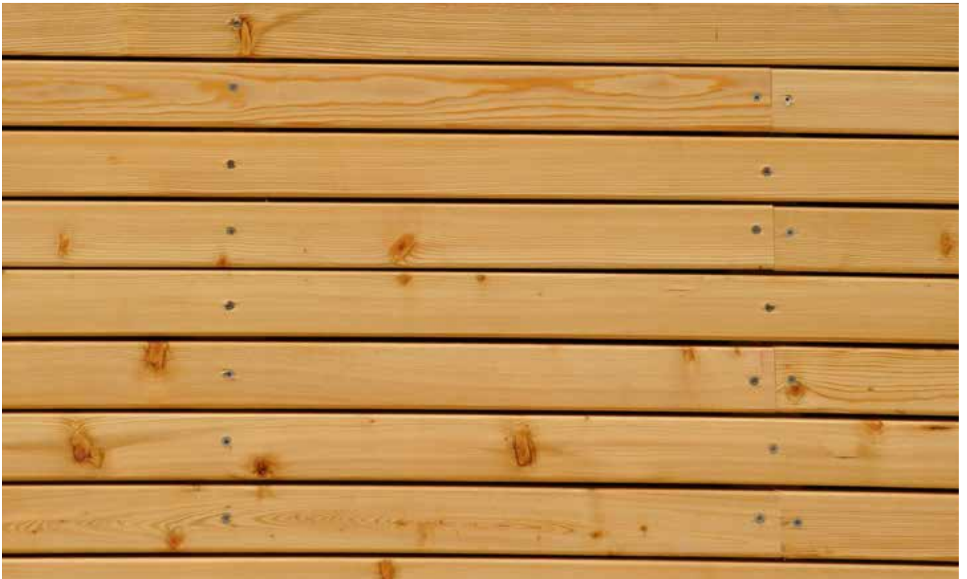
Detail of Raute profile 28 x 68 mm
